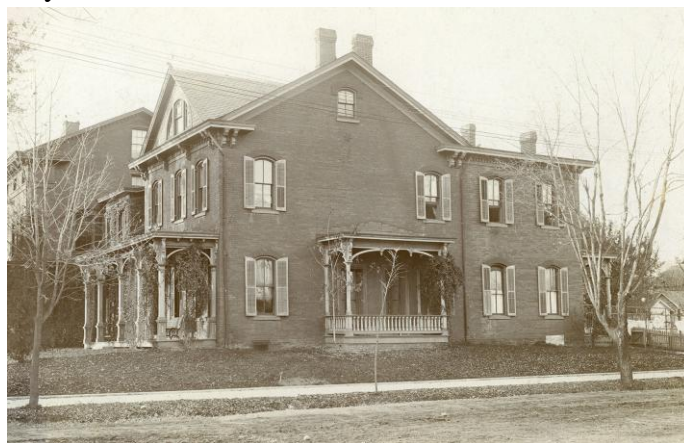
The second parsonage, seen here c.1900, was owned by the church for 54 years and is currently undergoing extensive remodeling.
