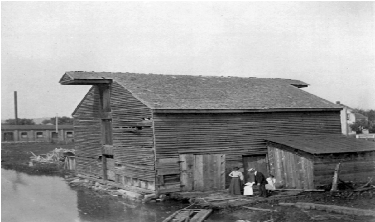
The McKelvy Warehouse on the north side of the North Branch Canal west of Market Street
