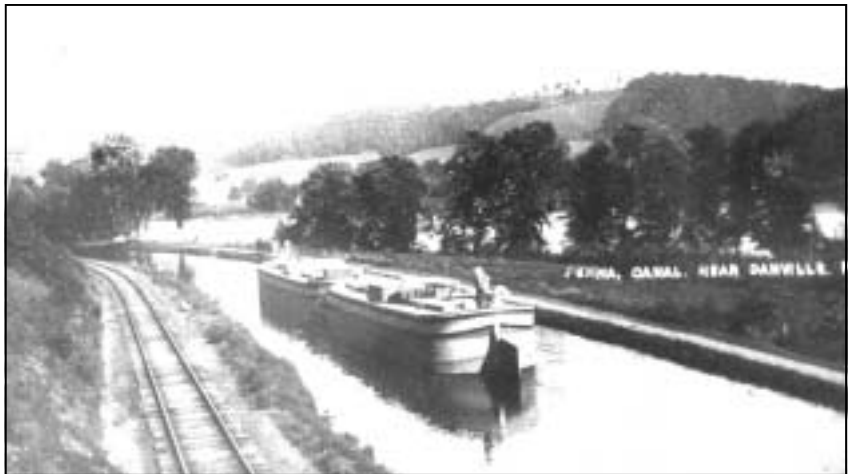
Delaware, Lackawanna & Western Railroad paralleled the North Branch Canal between Danville and Bloomsburg.
