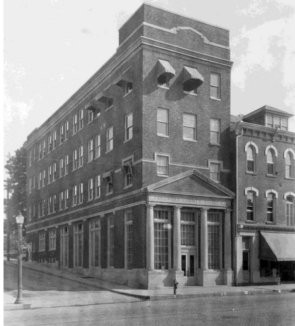
The Columbia County Trust Company building with its original entrance, c. 1920
